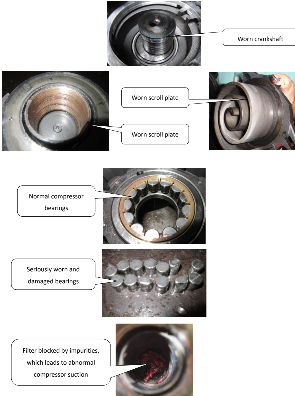
Figure 5-4.17: Effects of spoiled compressor oil
